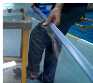
Step 2: install the Magnetic PVC strip on glass edge
