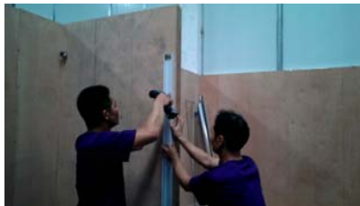
Step 4.Fix all the frames by screws.
