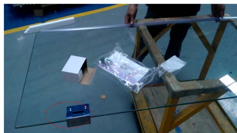
Step 1: Install 2pcs sus304 hinge on door glass
