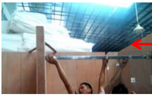
Step 5: open sliding rail holder, get out the screw and fix the rail holder to the 2-side of the wall on the position which we marked before.
