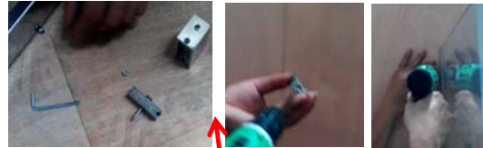
Step 5: open sliding rail holder, get out the screw and fix the rail holder to the 2-side of the wall on the position which we marked before.
