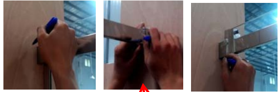
Step 3: mark the position of the rail on the wall
